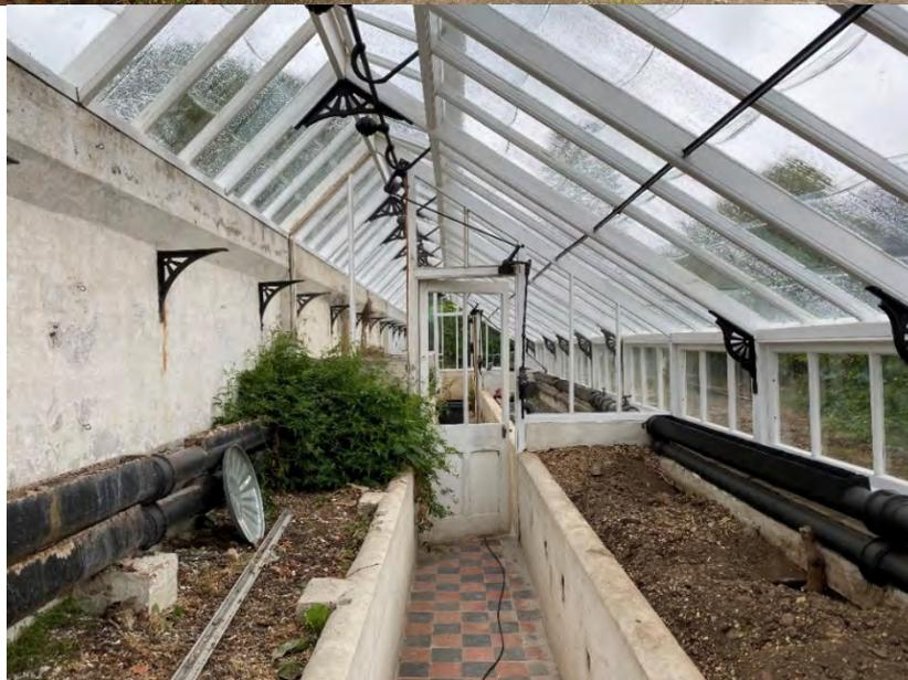
In this greenhouse all of the original features can be seen, the special glazing system, the iron work for opening windows and pipes for heating and humidification (these pipes can no longer be used as they were part of a much bigger system not in place anymore).
